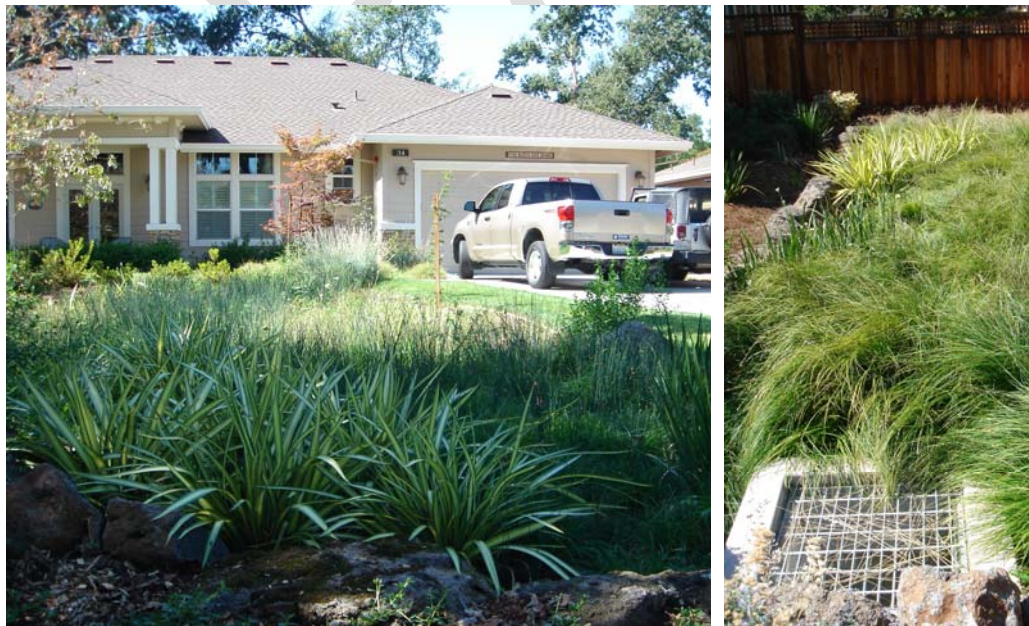
Figure 7.19a: Bioretention Systems within lots (front setback to house).Photos S.Boer (AECOM)
