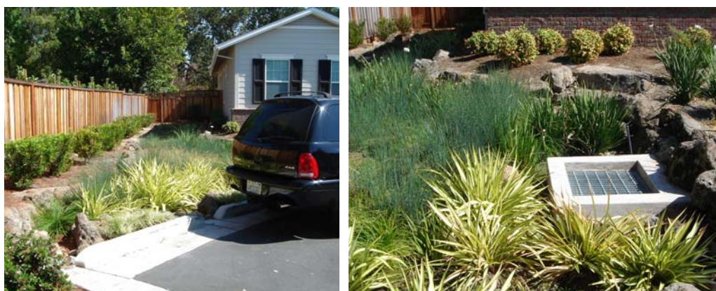
Figure 7.19b: Bioretention Systems within lots (front setback to house). Photos S.Boer (AECOM)
